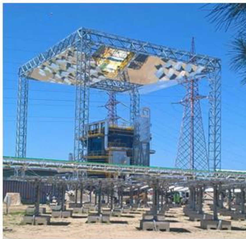
Example of new CSP technology: a solar accumulator integrated to a PV plant
